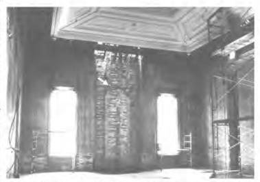
South Hall. University of California, Berkeley. During retrofit in the 1980s. Wall coverings and fireplace flue bricks have been removed. Horizontal pieces of bond iron can be seen running across the flue between tops and sills of the right and left windows. *Photograph by author.*
