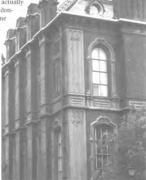
South Hall. University of California, Berkeley. Southeast corner illustrating pilasters which are fastened to bond iron and threaded rods by decorative nuts at the level of the window cornices on each floor. *Photograph by author.*
