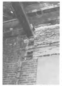
South Hall. University of California, Berkeley. During retrofit in the 1980s. Edge of vertical iron T column and iron girders exposed after wall excavation. Bond iron can also be seen in front of the T column. *Photograph by author.*
