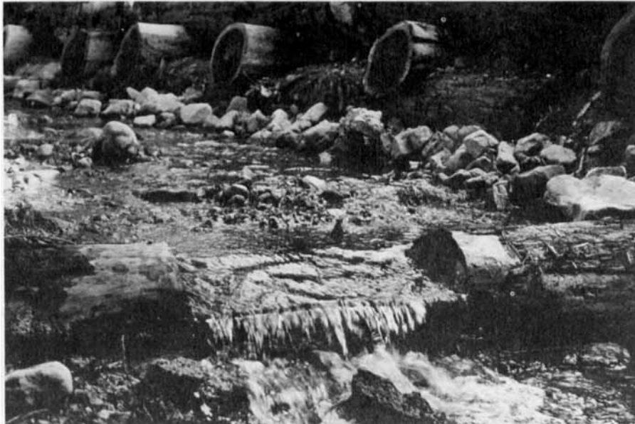
Figure 4. Notched redwood-log check dam in the creek.
