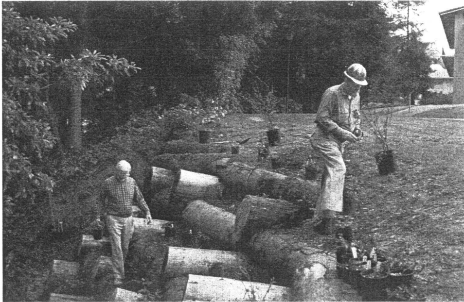
Plantings in cribwall. Courtesy of Vincent Resh.
