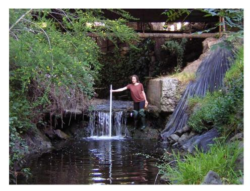
Figure 12. Down-cutting of streambeds below culverts has created most of Codornices Creek's fish barriers
