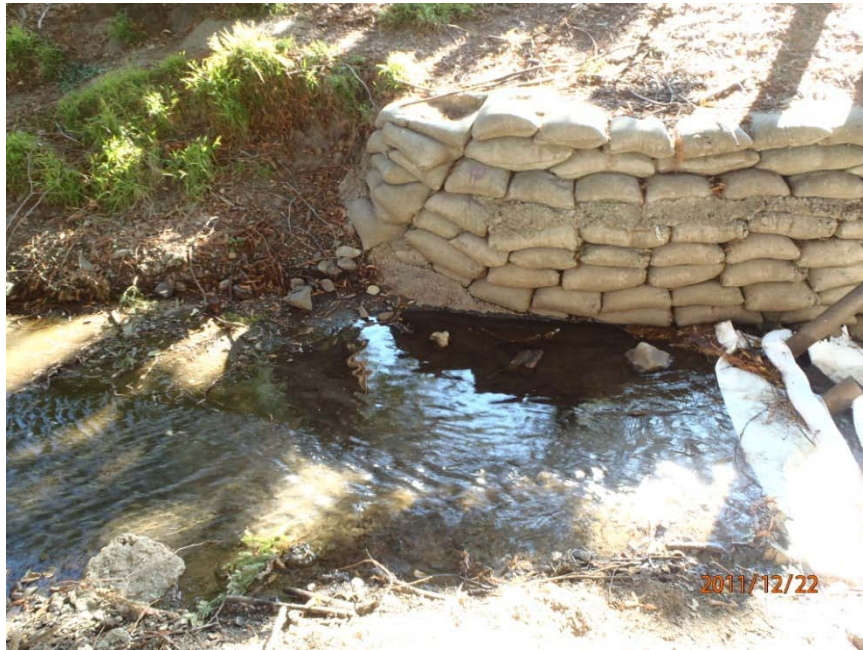
BK1-5 Water Sample Location upstream of Oxford Culvert
