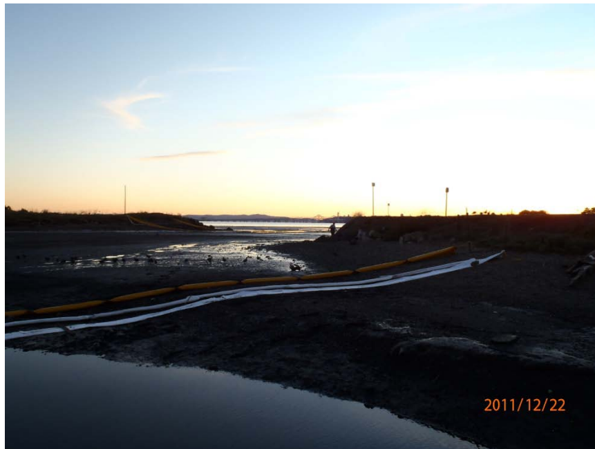
Looking at BK1-15 from BK1-14, Inside the Boom.
