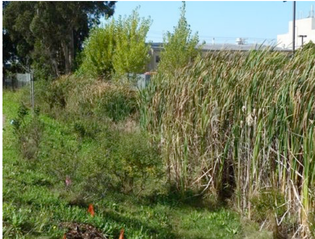
Photo 8. Typical channel conditions in 2011-excessive growth of cattails covering most of creek channel bottom (requiring maintenance to allow for creek channel flow.)
