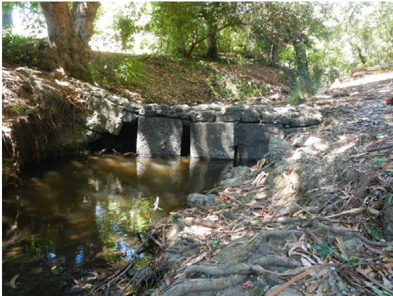
Photo 4: Check dam 2 (CD2) is about 35 feet upstream of CD1 on the North Fork. Notice instability on the right bank (left side of picture).
