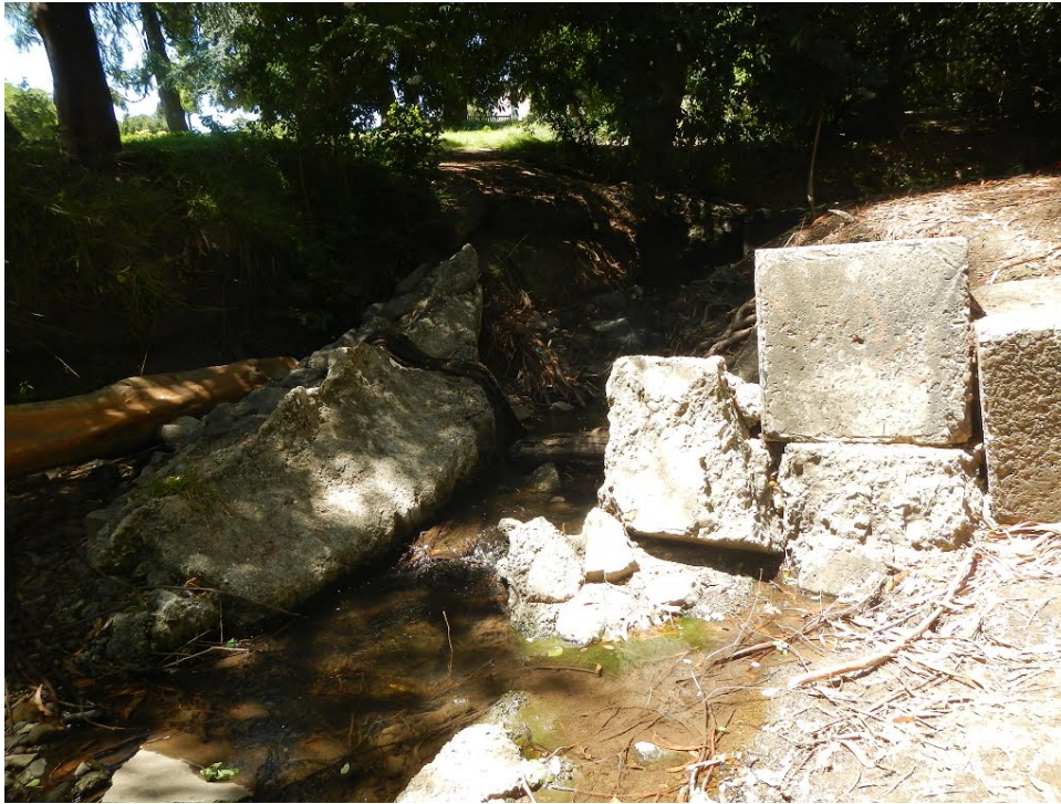
Photo 1: Failed check dam 1 (CD1) looking from the confluence upstream to the North Fork.
