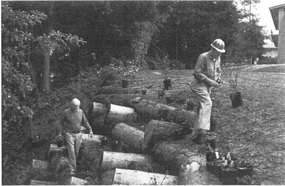
Plantings in cribwall. Courtesy of Vincent Resh.
