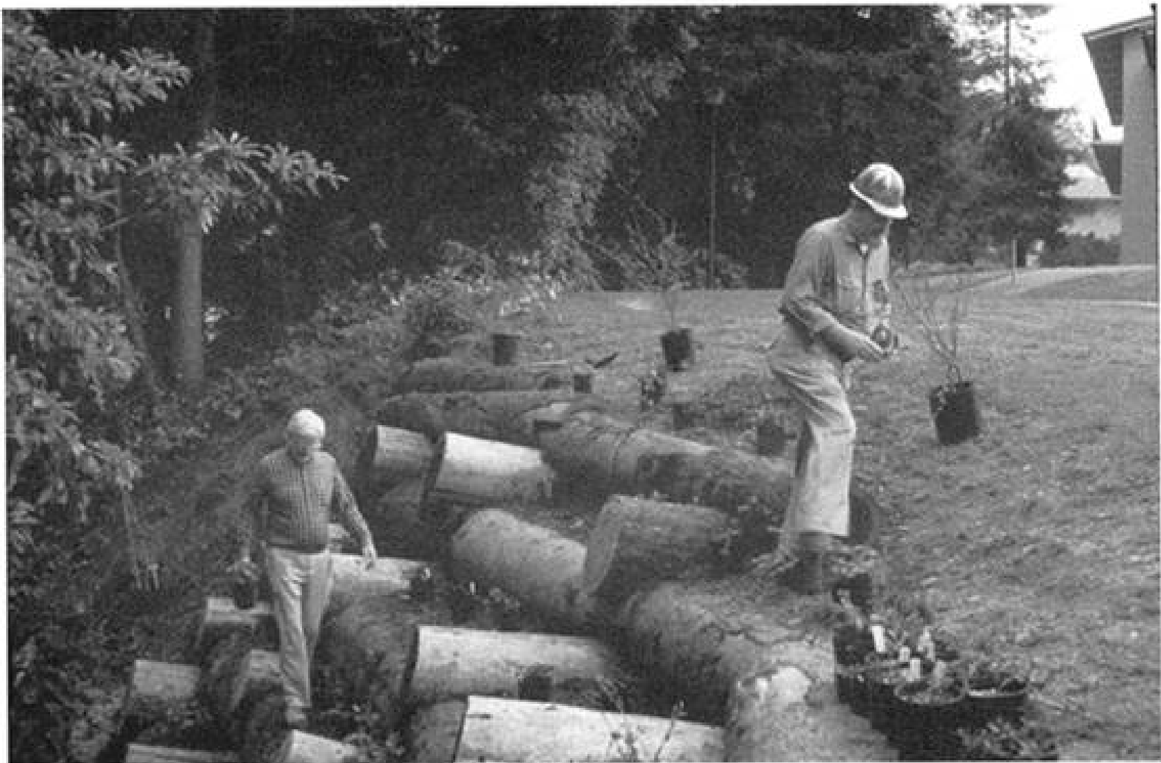
Plantings in cribwall. Courtesy of Vincent Resh.
