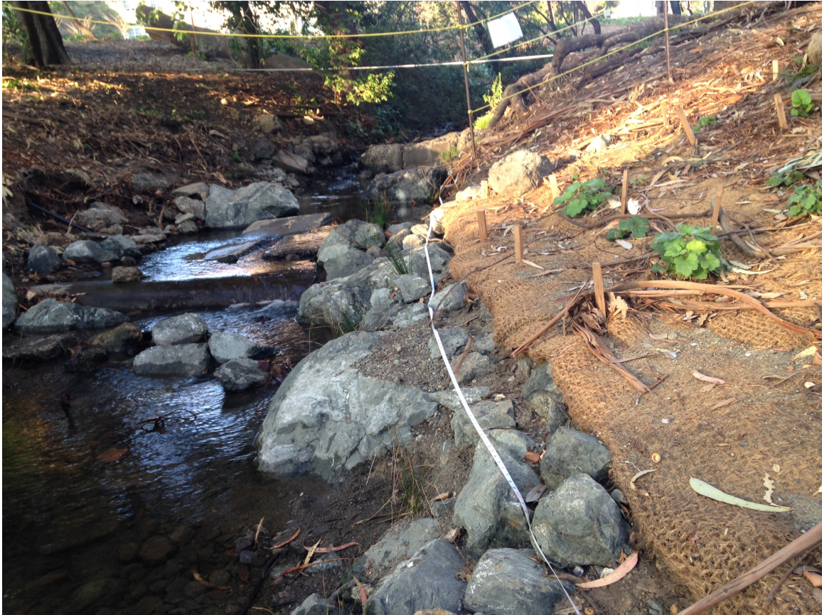
Figure 7. The restored section of the creek that was surveyed reveals a “step” change in elevation through the use of an embedded log (on the left, middle portion of the photo). The log works to break up energy received from the culvert upstream and also enhances the aquatic ecosystem by mimicking pools found in nature in this type of creek. The banks were stabilized with rocks of varying sizes and vegetation was planted along the banks with staked mats to decrease erosion as plants become established.
