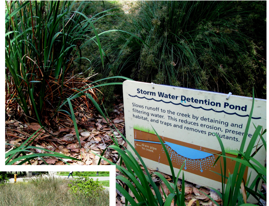
Above Left: An overflow drain from the grass biofilter carries runoff into the detention pond. Above: The detention pond filters and retains storm water before it flushes into the creek. Left: The detention pond is planted with native shrubs and grasses.
