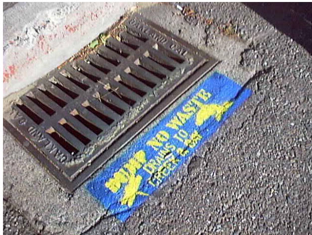
Example of Storm Drain Catch Basin Stencil
