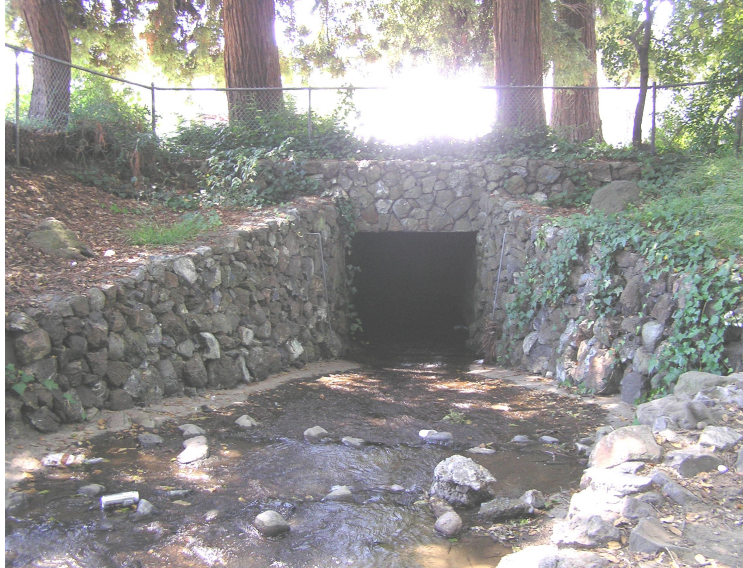
Oxford Street culvert during low flow
